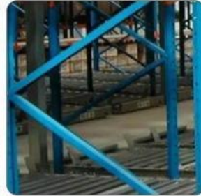
Inclined tie rod
